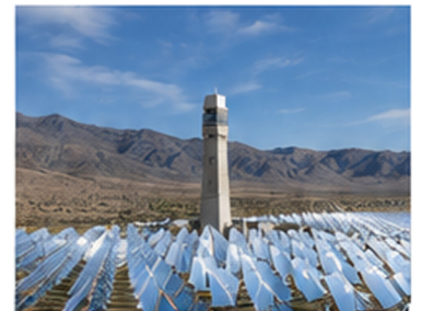
SOLAR THERMAL PLANT
