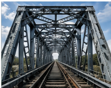
RAILWAY STEEL BRIDGES
