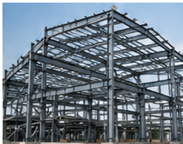
PRE ENGINEERED BUILDING
